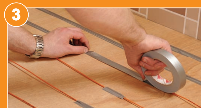
3 Apply adhesive tape over the entire length of the cable to secure in position.
