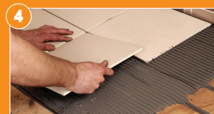
4 Apply flexible tile adhesive and lay the tiles.
