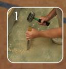
After preparing a smooth surface, measure the area to be heated and fit the insulated tile backer board to the floor securely following the manufacturers instructions. Create a groove in the board to accommodate the tubing for the floor probe.
