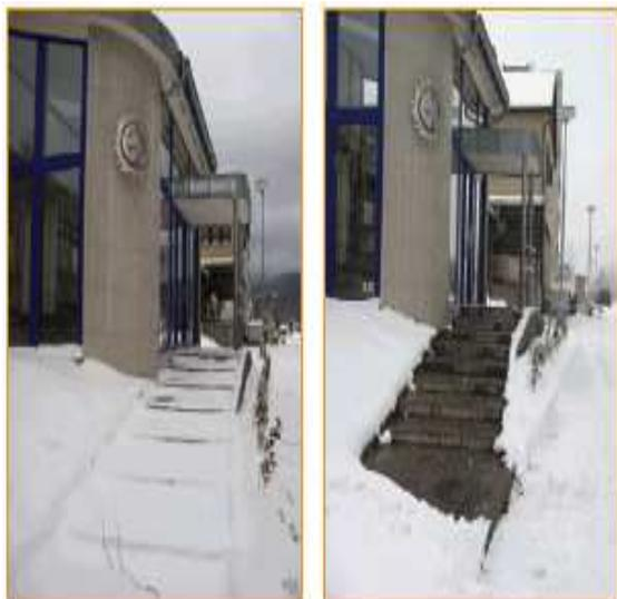
In the case of snow fall, an ice prevention system will quickly melt any snow that falls providing clear, access for pedestrians and vehicles on pavements and drives.
